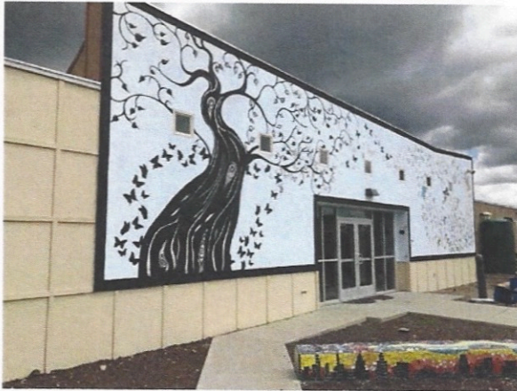
Looking NE – Building 1 Exterior
