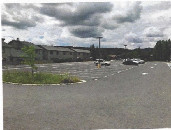
Typical Open Parking Spaces
