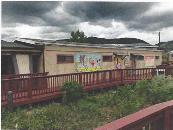
Looking NE – Building 6 Exterior
