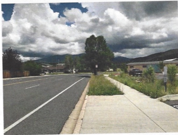
Looking N – Fremont Boulevard ROW
