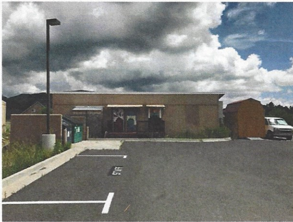
Looking E – Building 8 Exterior
