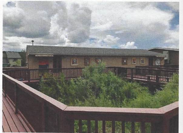
Looking SW – Building 5 Exterior
