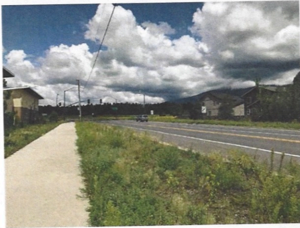
Looking NW – Fort Valley Road ROW
