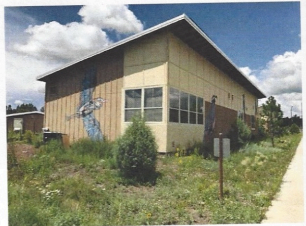
Looking SW – Building 1 Exterior
