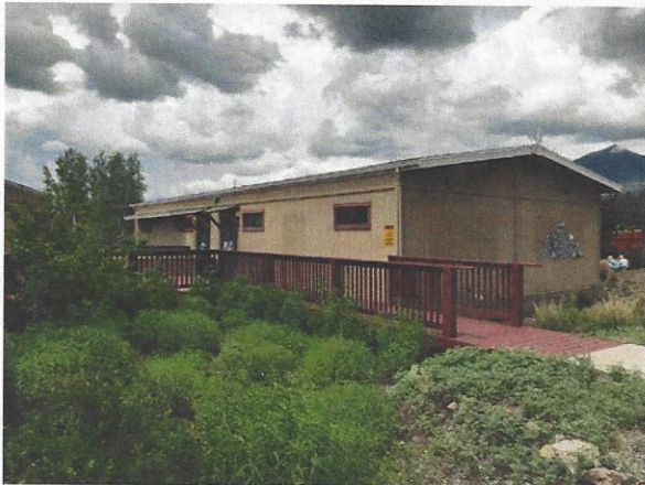
Looking NW – Building 2 Exterior
