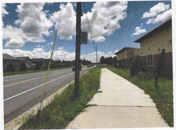
Looking SE – Fort Valley Road ROW
