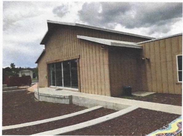
Looking NW – Building 1 Exterior
