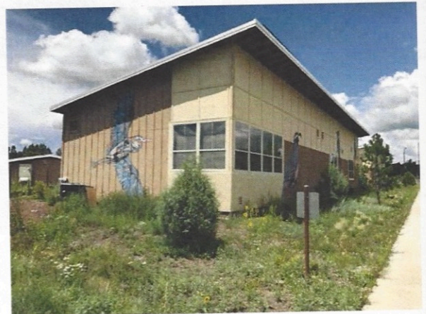
Looking SW – Building 1 Exterior
