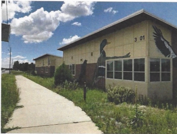
Looking S – Building 1 Exterior
