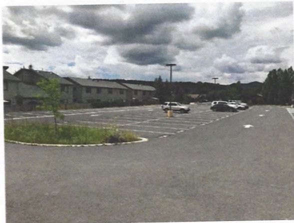
Typical Open Parking Spaces
